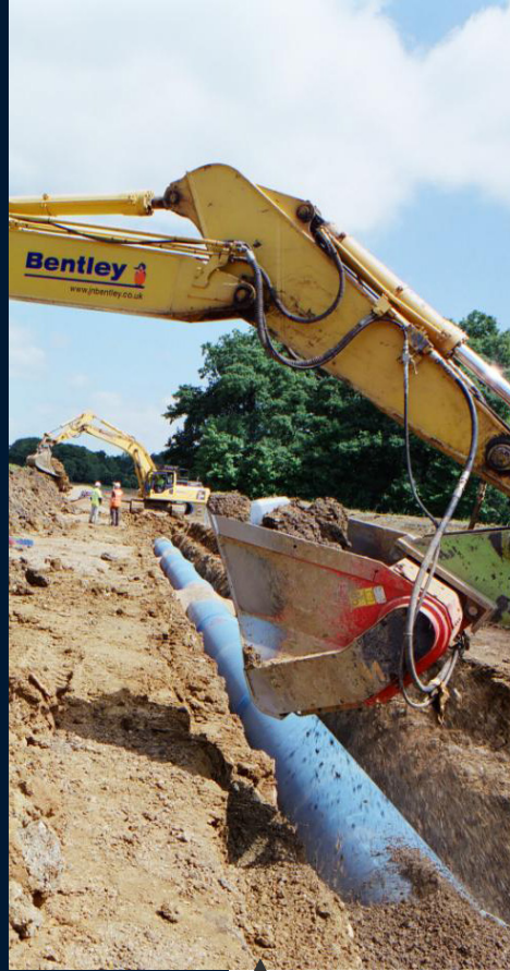
2000: Construction along the Wing Pipeline.
