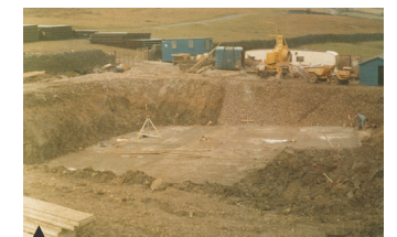
1976: Excavation for Reeth service reservoir.
