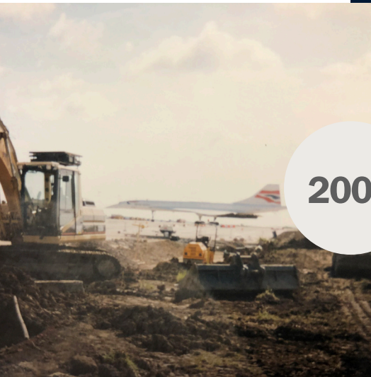
2001: Clay lining a new area prior to landfilling at Skibeden just outside Skipton.
