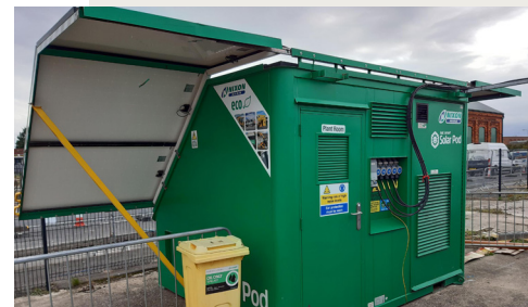
Solar smart site set-up.
